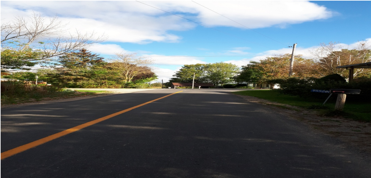
Canning Road approaching Township Road 3 from the South. Blind corner if making a right hand turn.
