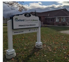
New exterior signage installed at the Princeton Branch
