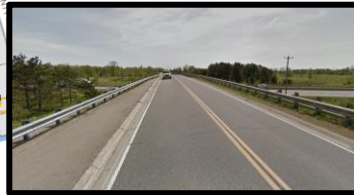
County Road 29 at Highway 401 Overpass crossing
