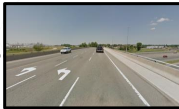
County Road 10 at Highway 401 Overpass crossing
