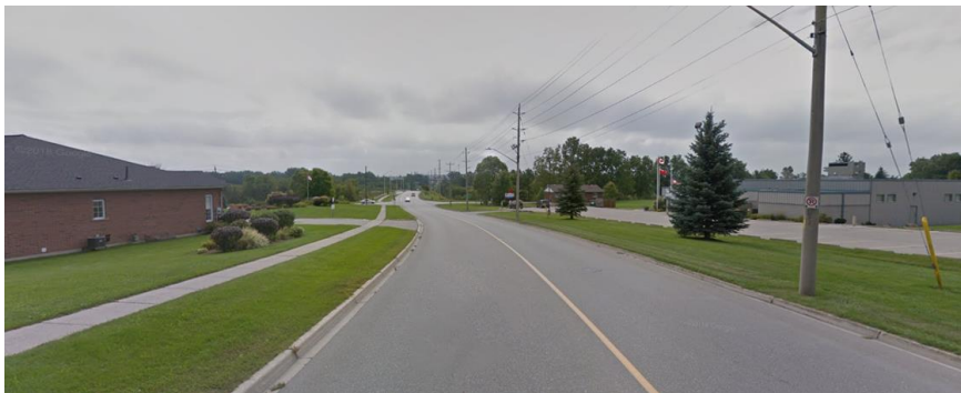
Ingersoll Street / County Road 10
