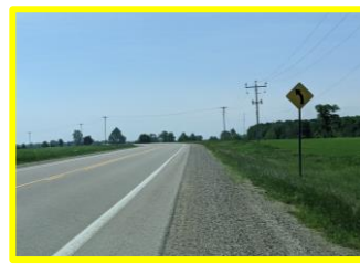
Partial paved shoulder and gravel shoulder
