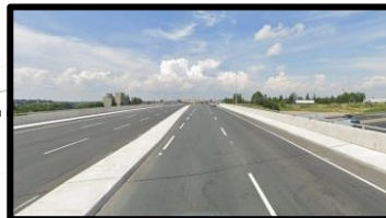
County Road 59 at Highway 401 Overpass crossing
