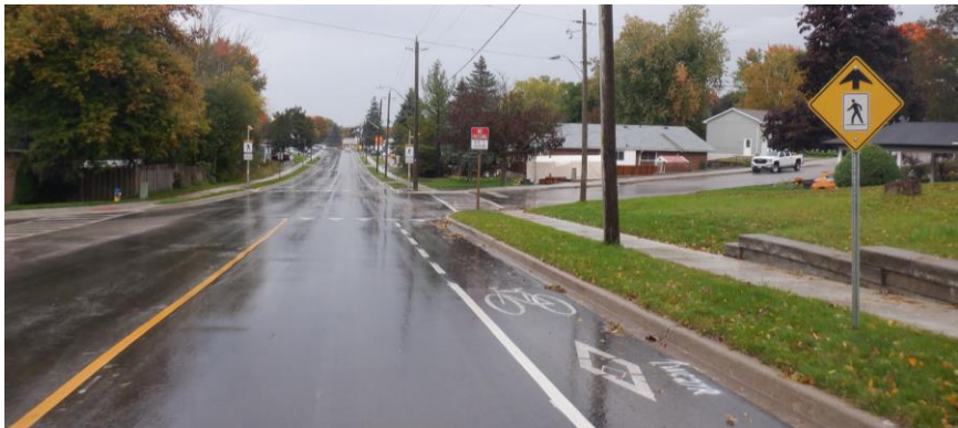
County Road 119 / Bell Street
