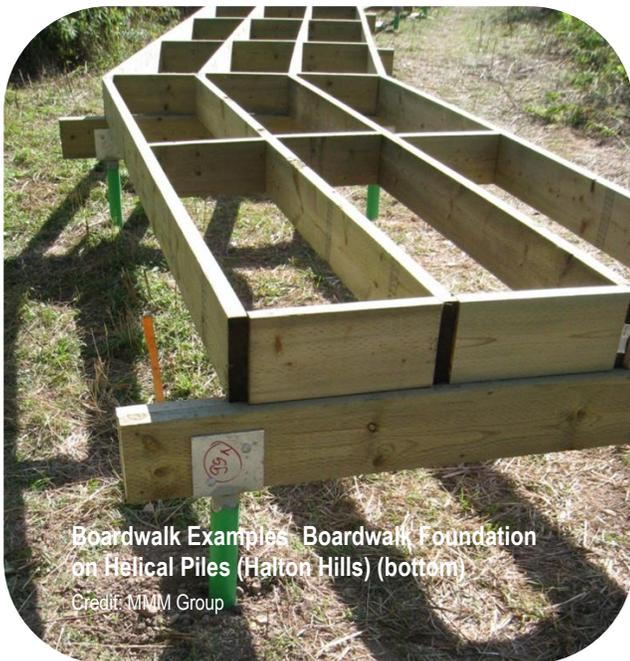
Boardwalk Examples - Boardwalk Foundation on Helical Piles (Halton Hills) (bottom)
