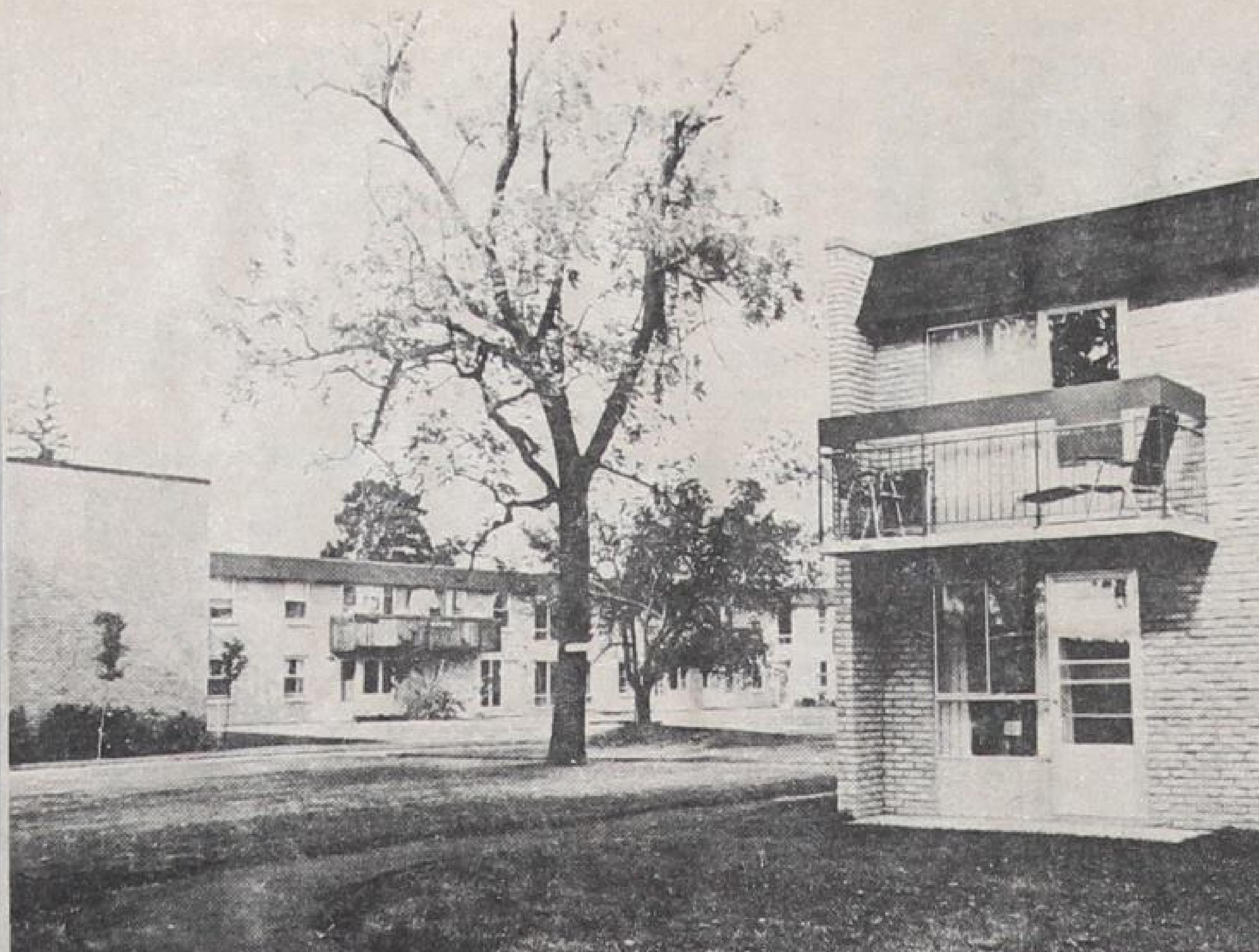
A typical setting of Ontario Housing Corporation's senior citizen complex. Each one bedroom apartment comes equipped with stove and fridge in the kitchen. Each has a living room with small patio or balcony (Ministry of Housing photo).
