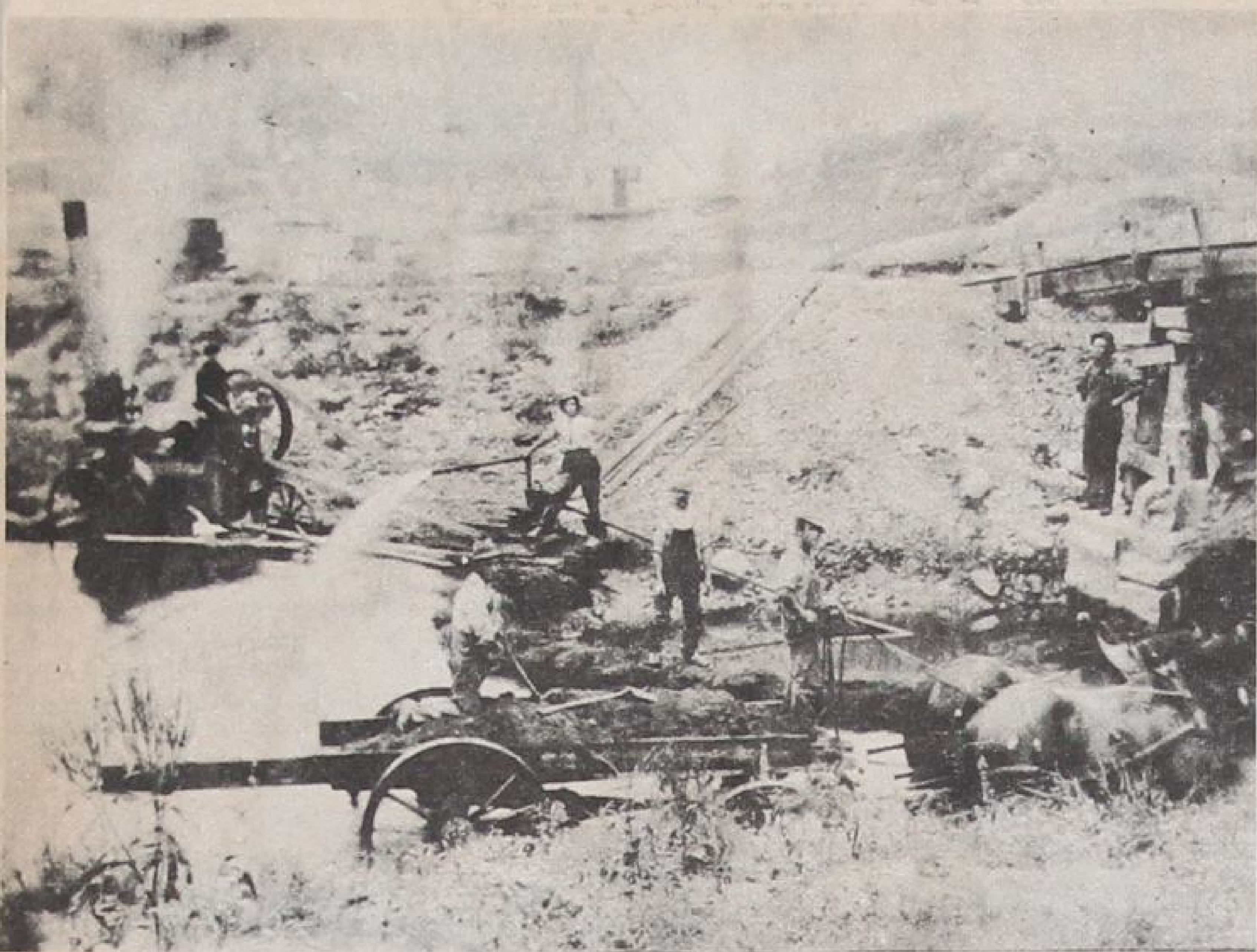
As shown above in this 1907 quarry scene, operations were primitive and workers had to go to great lengths to obtain limestone from the water-filled pits and transport it to nearby kilns for burning. In those days before modern technology, limestone was measured in bushels.
