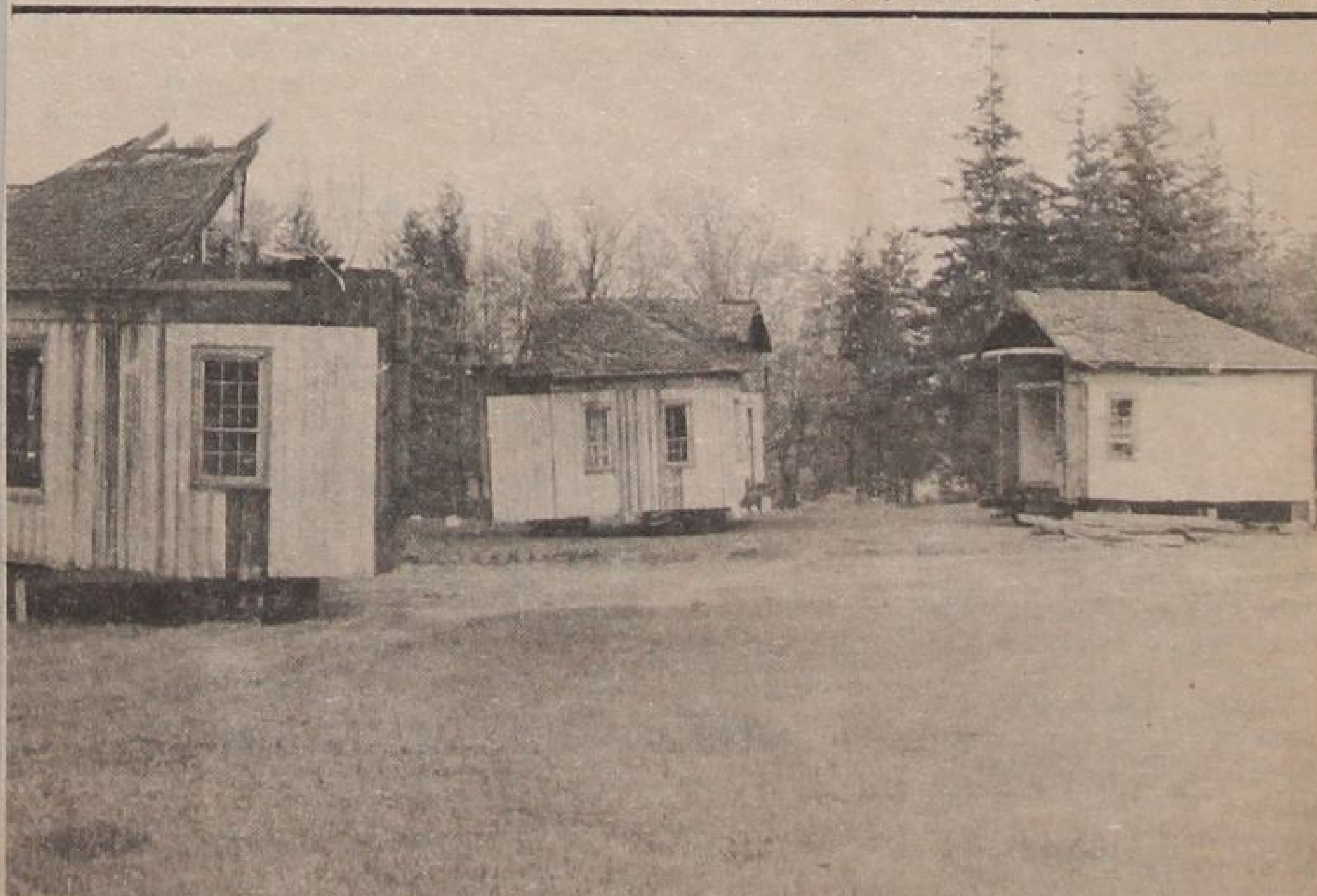
The Oddy house, originally located just south of Milldale on 59 Highway now sits in three pieces on movers equipment at its new site, donated by Norwich Township, at the west end of Otterville. The project to save the rare, octagonal-shaped house is spearheaded by Mrs. Don Pettigrew of RR 1, Otterville.
