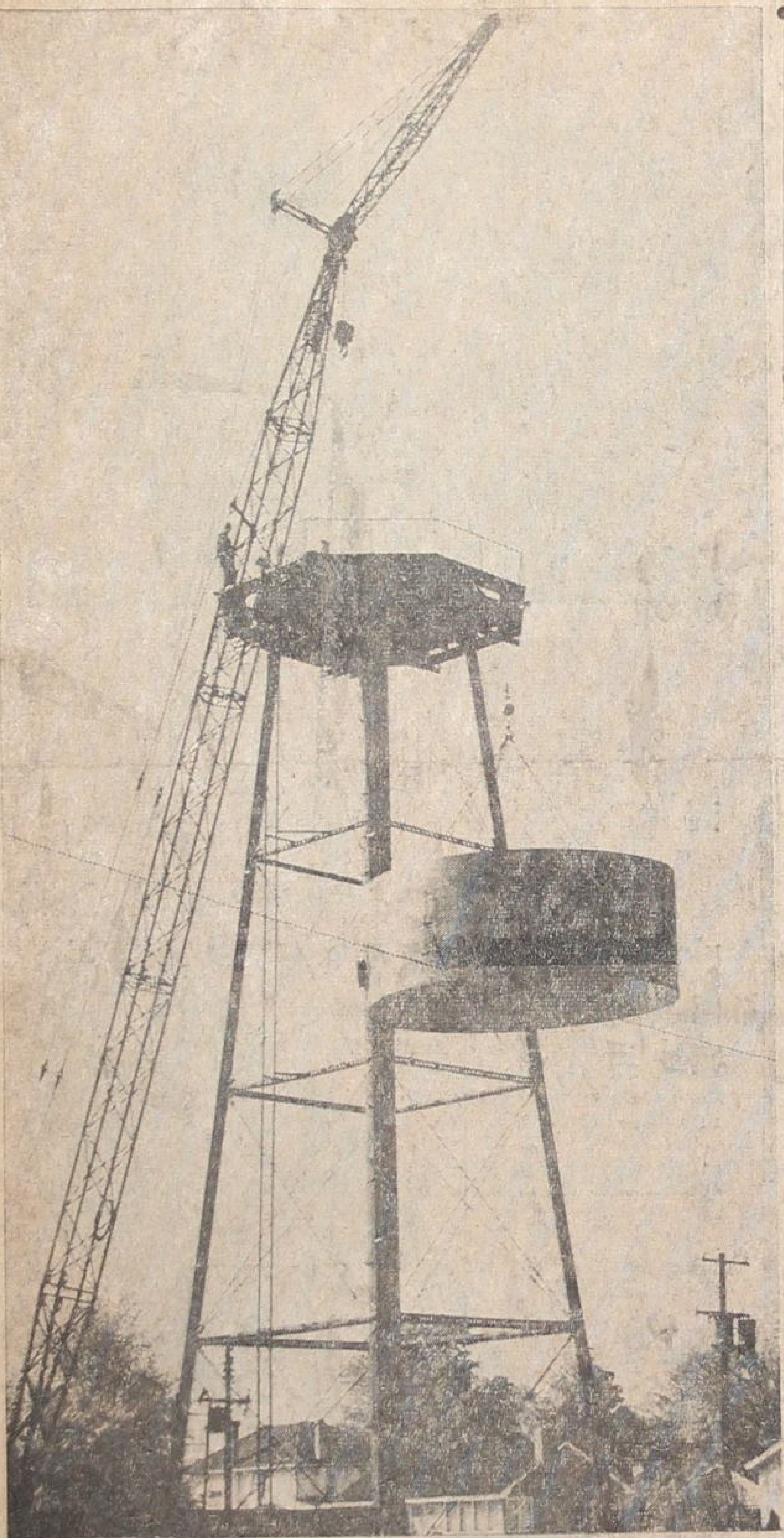
Erection of a new tank to service Otterville's water system was underway last week. The first section, shown here is being raised by a 110 foot derrick owned by Bridge and Tank Company of
