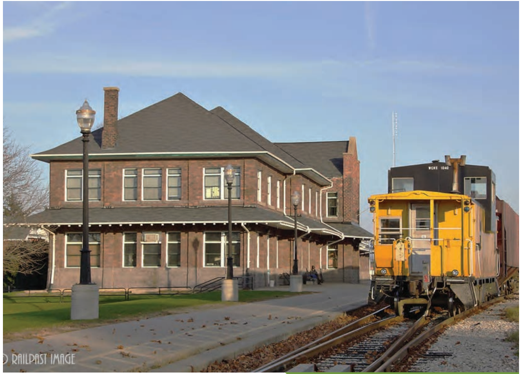
The Georgetown-London Guelph Subdivision requires a progressive program of upgrading to decrease running times and allow for SouthwestLynx frequency increases. The extensive sections of jointed rail, the rail fasteners, the ties and much of the underlying substructure need to be replaced to provide a smoother and faster ride. Photo by Walter E. Pfefferle
