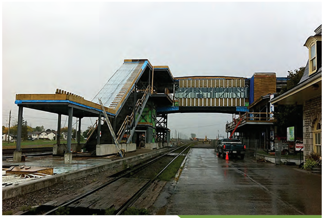
In addition to adding a third main track at the stations listed above, a far-side platform and a fully-accessible passenger overpass will be required, as VIA constructed at certain points along its Toronto-Montreal route.
