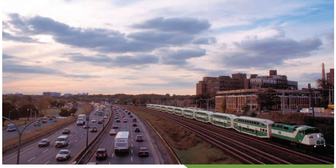
A four-track railway line can handle the passenger and freight equivalent of 32 lanes of highway traffic. Creating this highway capacity would rip a jagged wound through any urban or rural area, while the existing rail corridors can usually accommodate additional tracks with little or no extra land. Photo by Tim Hudson
