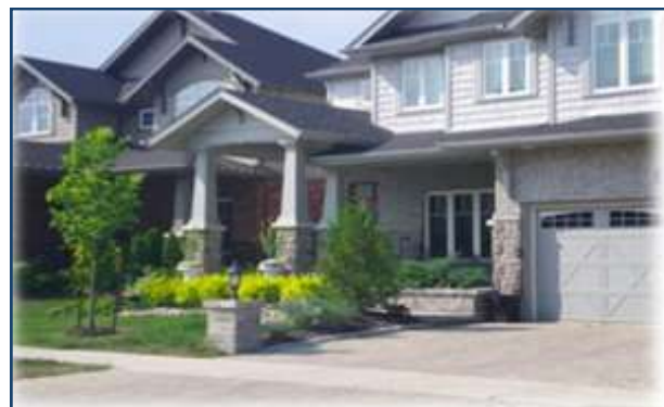
Garages that are flush with the house place the emphasis on the porch and front door instead of the garage. architectural treatment of garage doors is encouraged.
