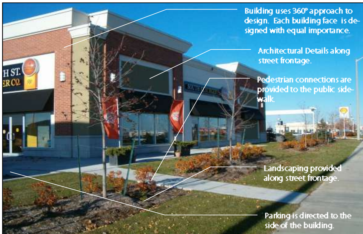
While more of an urban example, the above photo illustrates elements of good commercial design.
