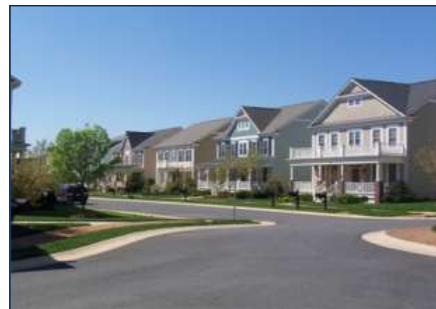
Streetscapes are enhanced by providing a variety of architectural treatments including porches, peaked roofs, dormers and various window shapes/sizes.
