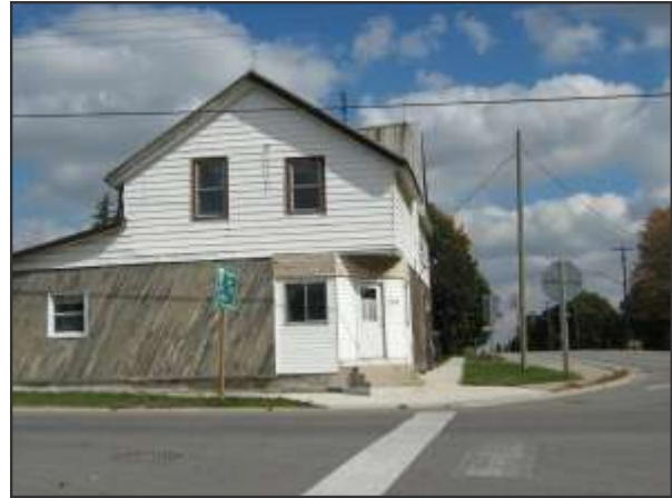
Building close to street line at main intersection
