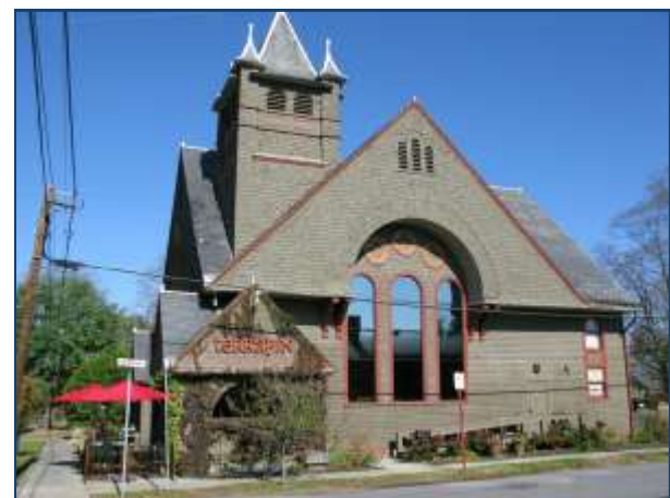
Adaptive re-use of former institutional buildings is encouraged, particularly in the Village Cores.
