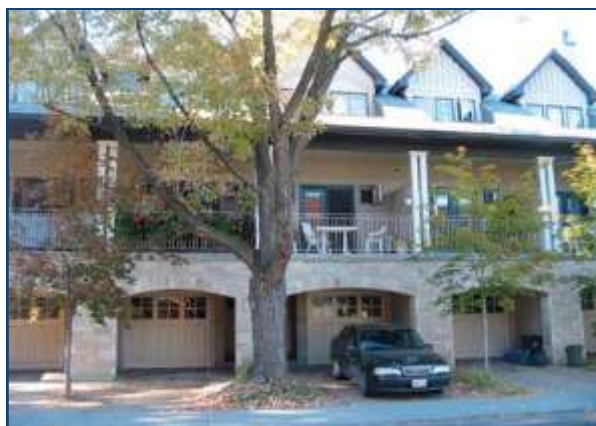
Depending on the grade of a site, parking may be provided below residential units at the rear of a site.
