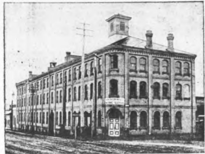
Head Office and Factory, Situated on Corner of Bain and Colborne Streets,
