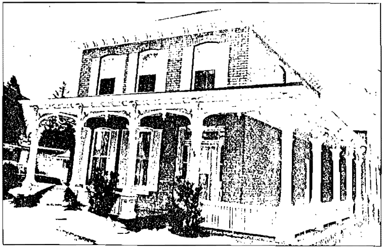
The Robins' home, built between 1850 and 1860, is very solid structurally and has seen a great deal of activity in its lifetime.
