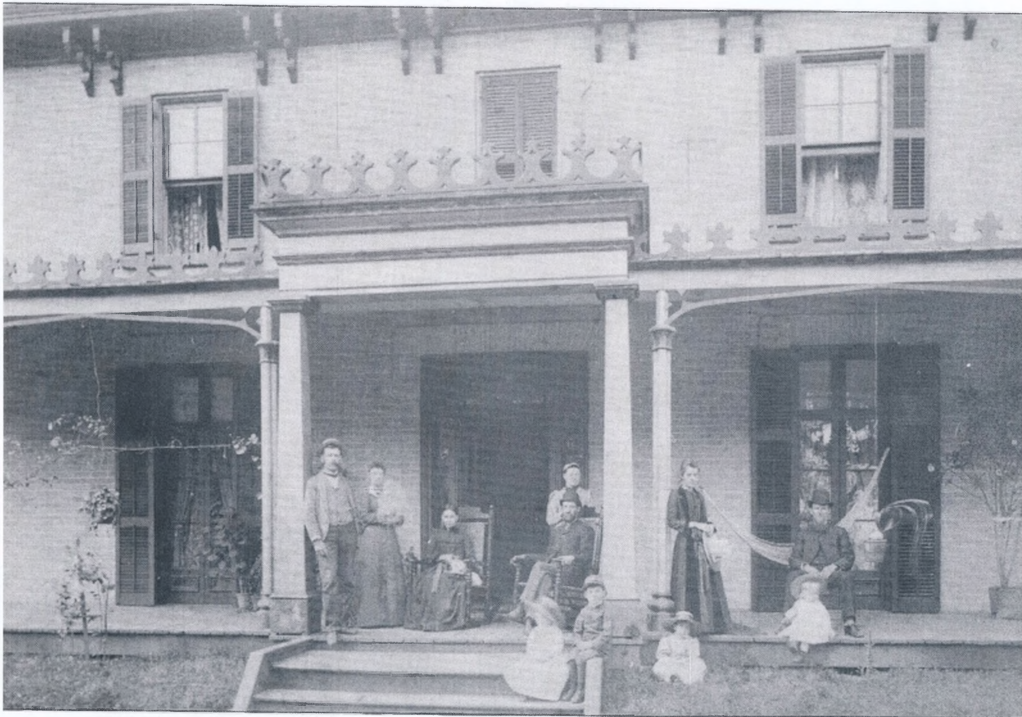
HOME ON EARL STREET, INGERSOLL
