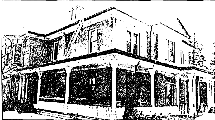
Work had to be done on the outside of the Simpson residence as well as the inside.
