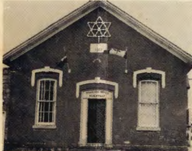
Beachville Municipal Office Built 1867
