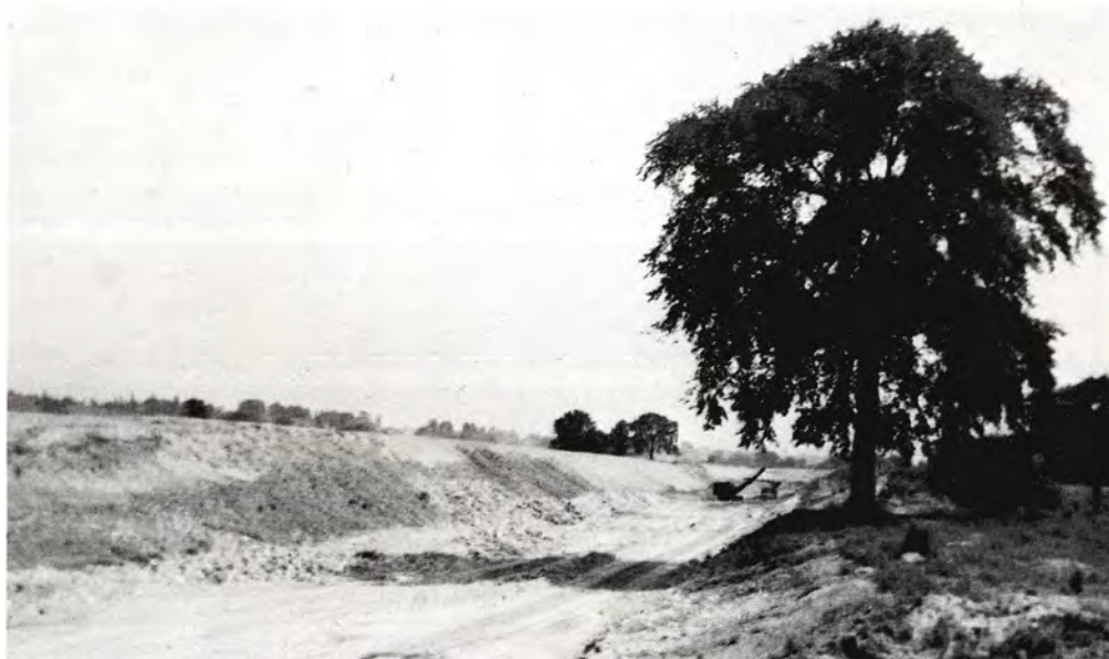
Digging new river channel, 1949. Elm trees are now all dead of elm disease.
