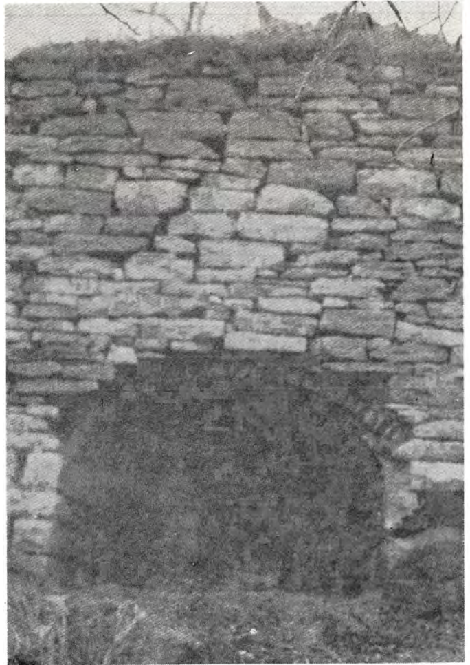
An old kiln showing portal for removing lime. Many of these kilns were in existence 75-100 years.
