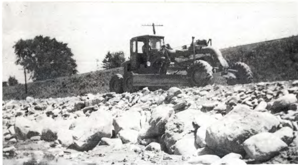
Digging new canal for the Thames, 1949. Bumpety-bump-bump! Copyright by M. Cropp, Beachville, Ont.
