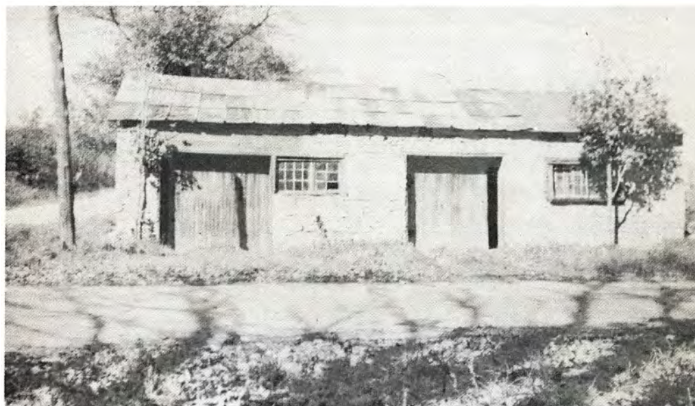
Remains of Burdick's Furniture Factory, destroyed by fire, were roofed and used as a blacksmith shop.
