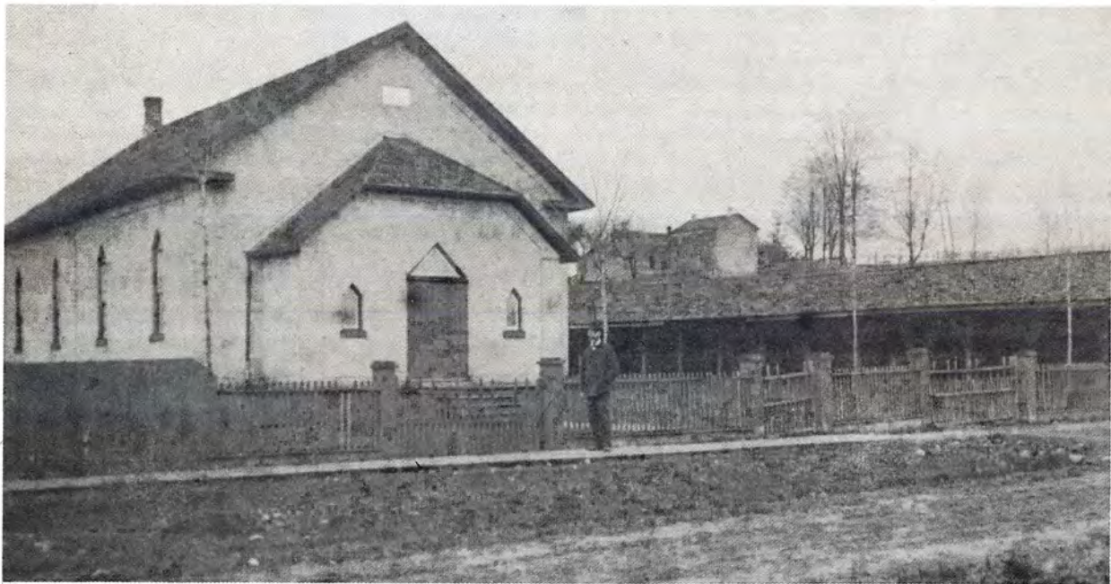
Baptist Church - burned 1943. Erected in 1866.
