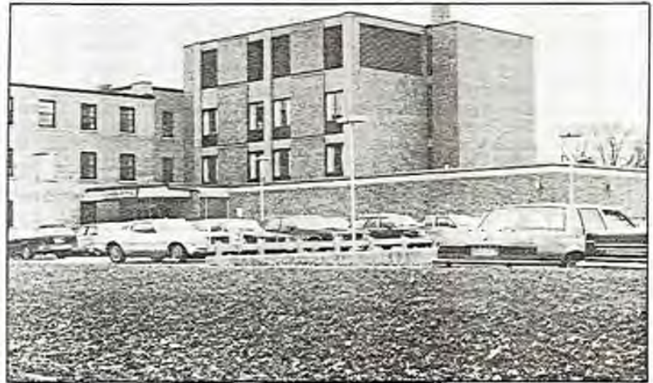
The 1970 addition included the ground floor emergency area and a third storey. For two years, the hospital ran its own ambulance service from this area.
