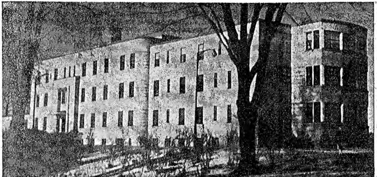
THIS IS INGERSOLL'S Queen Alexandra Hospital, built in the 1940's for $275,000 to replace the original structure erected in 1909 and named for Queen Alexandra. There were 1,911 admissions last year, and hospital officials see continued growth in the future as steps are taken to provide for many new forms of treatment.
