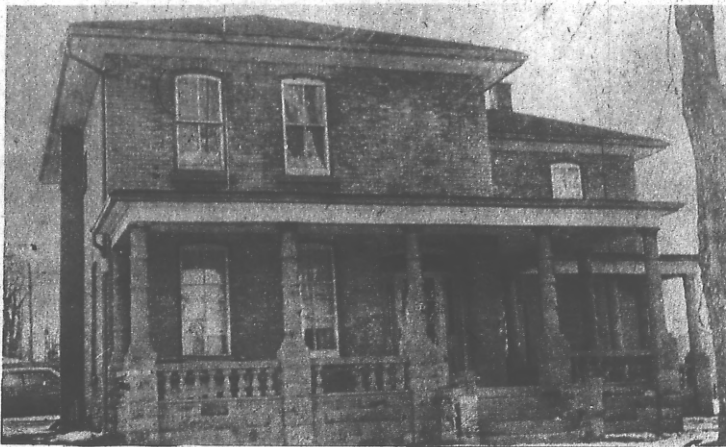
This house is located on the corner of McKeand Street and Victoria Street .
