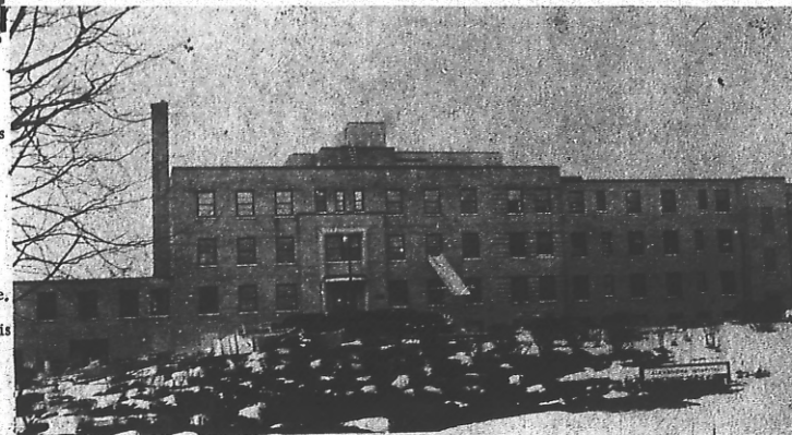
This is the site of Alexandra Hospital with expansion presently going on at the rear .
