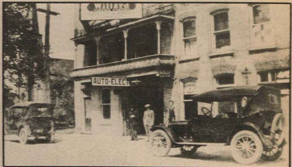
Fleischer & Jewett's 1920 location next to old Skinner building on Charles West at the bottom of Oxford Street in Ingersoll.
