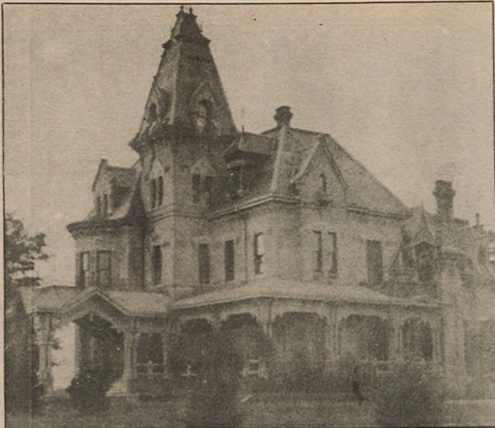
The former James Noxon home was the first Alexandra Hospital. A parking lot, and a portion of the present hospital are located where the house once stood.
