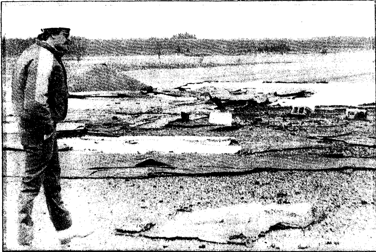
THE ROOF at Cobi Foods Inc. west of Ingersoll took a beating during heavy winds Wednesday night. Here, maintenance manager Tom Masson inspects the damage. Insurance adjusters were on the scene Thursday.
