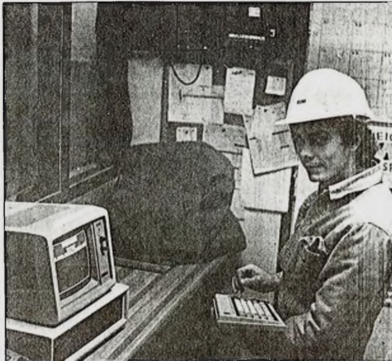
Craig Hutchison is one of two computer operators in the fertilizer division of Coldsprings in Putnam. The computer automatically controls every aspect of production, almost totally eliminating the human error factor.
