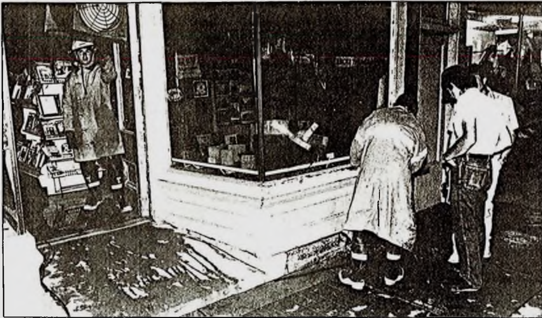
Firemen examine the damage at Carr's Book and China Shop Saturday night. The fire started in the front display window, quickly filling the store with smoke. Fire Chief Ken Campbell later estimated $1,500 damage was done to the building.
