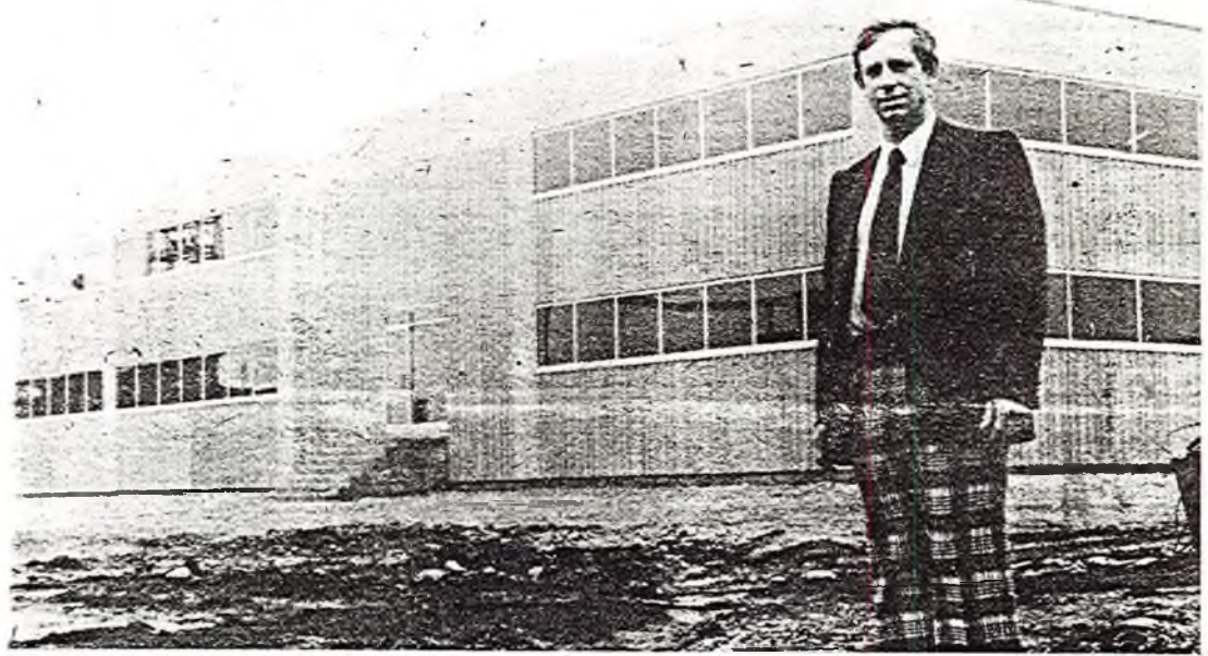
Ernie Wilson, general manager of Ingersoll Machine and Tool, sees an improved work environment as one of the major benefits of the company's $2-million expansion program.
