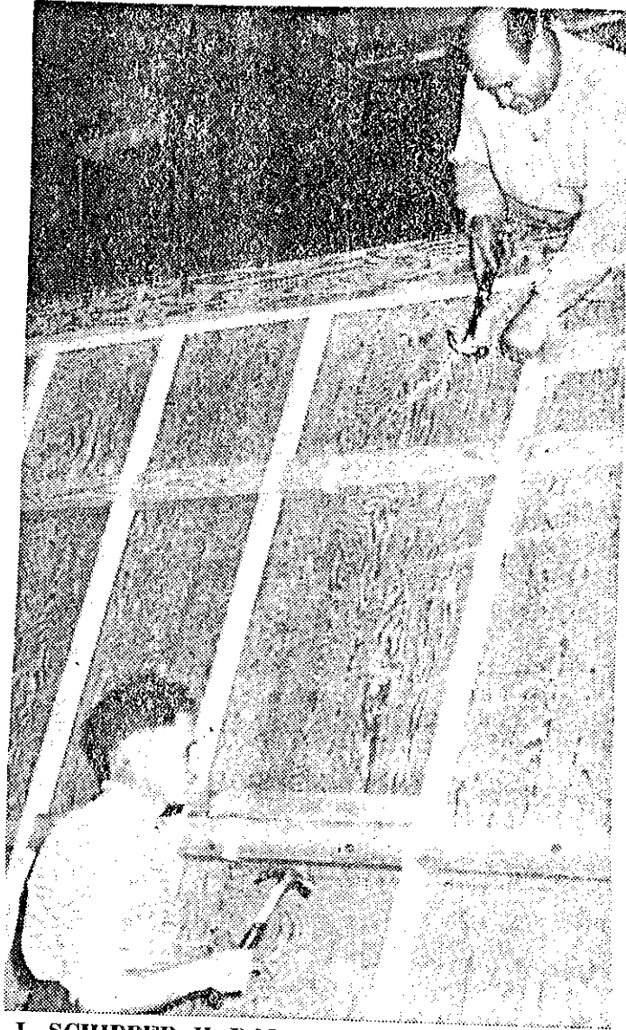
L. SCHIPPER, H. DAWDRY ASSEMBLE PANELS
