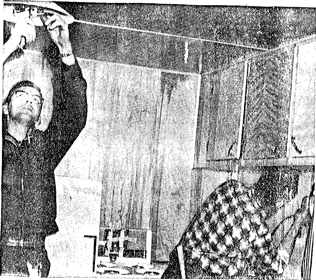
P. CLARKE, H. DAWDRY INSTALL INTERIOR FIXTURES
