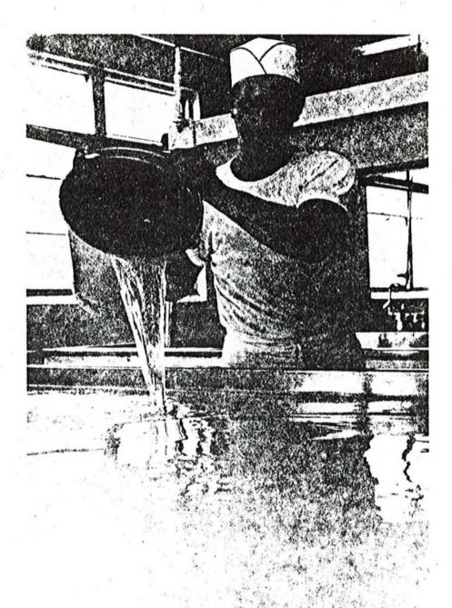
When the vat is full and the temperature reaches  $86^{\circ}F$ , rennet is added and the stirring stopped. If colored cheese is to be made, the color is added before the rennet. After coagulation, the curd is cut vertically and horizontally, leaving it in  $^{1}/_{4}$ -inch cubes. Immediately after cutting, gentle stirring again takes place. Contents of the vat are slowly heated to about  $100^{\circ}F$ .
