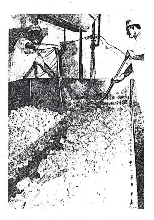
During the cooking or heating process, whey is expelled from the cubes and they shrink. We now have the commonly referred to mixture of "curds and whey". The cooking stage of cheese-making extends over a period of about 2 hours. Chemical changes take place, the acidity of the whey increases, the curd particles become firm, and then the whey is drained off. In this picture the curd is being piled, allowing whey to escape.
