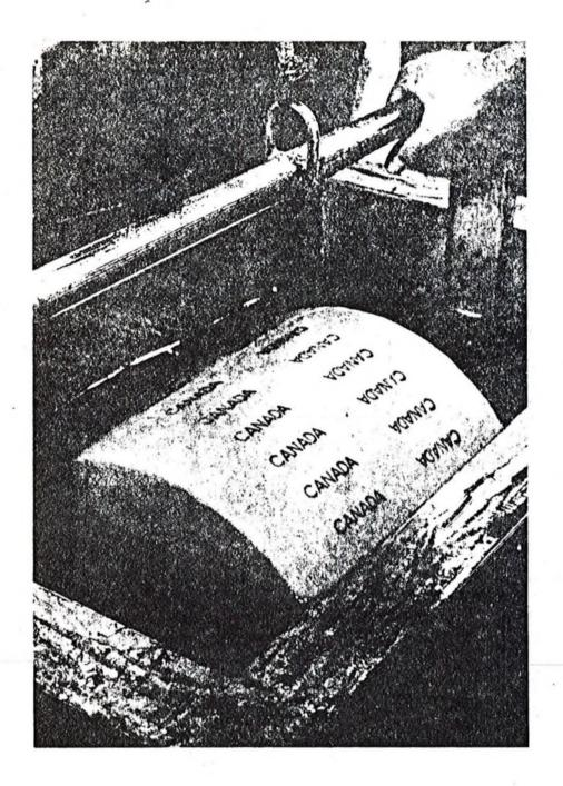
After the cheese has remained on curing room shelves for a number of days, the rind becomes dry and the cheese is ready for waxing. This is done by dipping the cheese in a tank of liquid wax at a temperature of approximately 240°F. Waxing prevents loss of weight, mold development and thickening of the rind.
