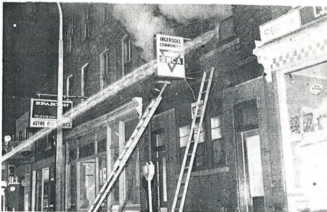
Extensive damage was done to the Y. M. C. A. by a fire early Saturday morning when the upper floor was swept with flames. Firemen had the fire under control but not before the whole building suffered from smoke and water damage.
