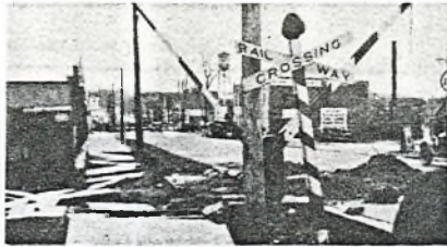
Sidewalks looking south on Thames Street that were ravaged by the April 1937 flood. (Photo by Doug Carr)
