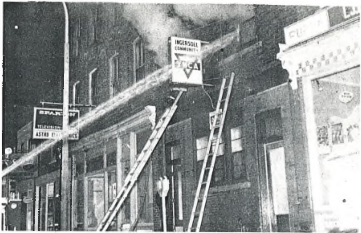
Extensive damage was done to the Y. M. C. A. by a fire early Saturday morning when the upper floor was swept with flames. Firemen had the fire under control but not before the whole building suffered from smoke and water damage.
