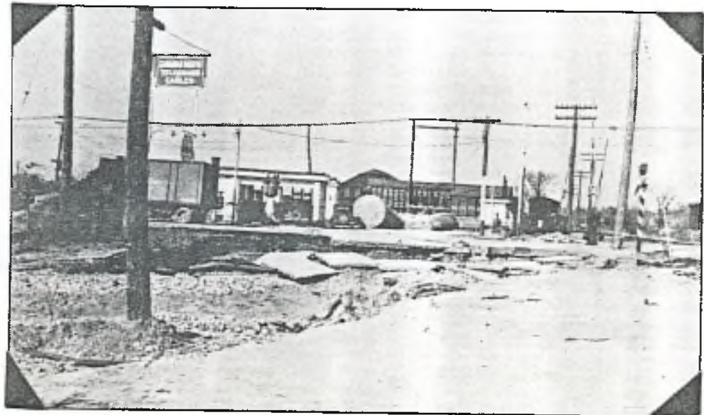
This photo, taken at the time of the 1937 flood, shows the Thames Street footbridge and some of the debris left on the banks of the river by the rushing water.
