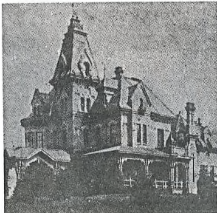
The old Alexandra Hospital, former home of industrial magnate James Noxon, was Ingersoll's centre of healing from 1909 to 1951 when it was moved into the building it now occupies.
