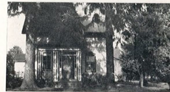
C. E. MERRILL RESIDENCE
