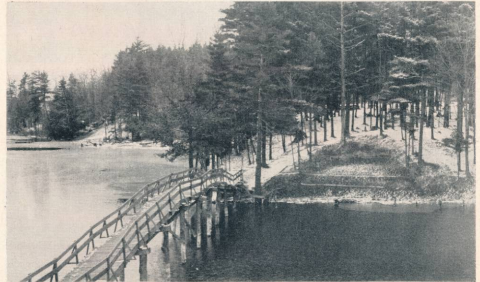
First Footbridge to Park
