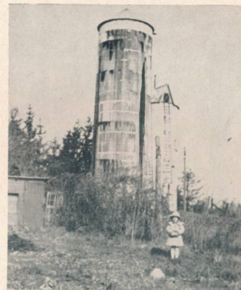
Old Water Tower
