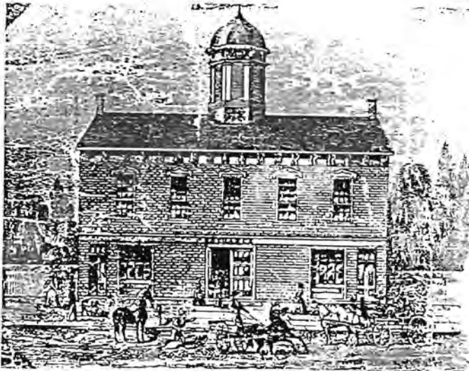
Original Market House & Town Hall
