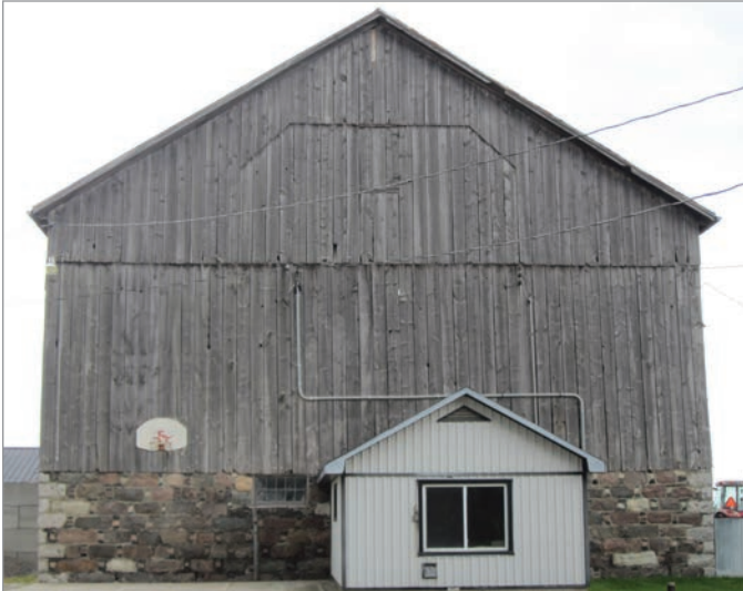
FIG. 18. CRELLIN'S ABERDEEN BOND BARN FOUNDATION, 13TH LINE, NO. 6332, OXFORD COUNTY. | KAREN E. ARMSTRONG.
