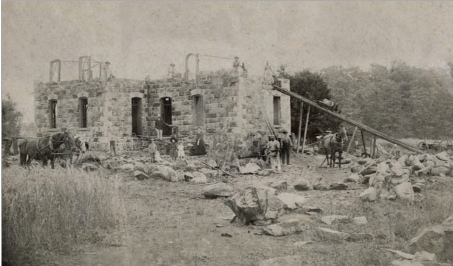
FIG. 20. ALEXANDER SUTHERLAND HOUSE, CONSTRUCTION SITE, 1891, ROAD 74, NO. 4358, GOLSPIE, OXFORD COUNTY. | SPECIAL THANKS TO KEN JUDGE.
