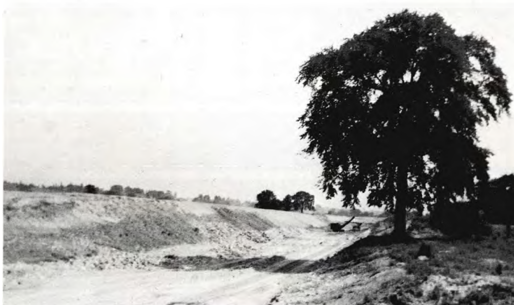
Digging new river channel, 1949. Elm trees are now all dead of elm disease.
