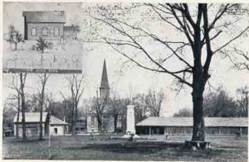
FRAME CHURCH ("AULD KIRK"), AND MEMORIAL PARK
