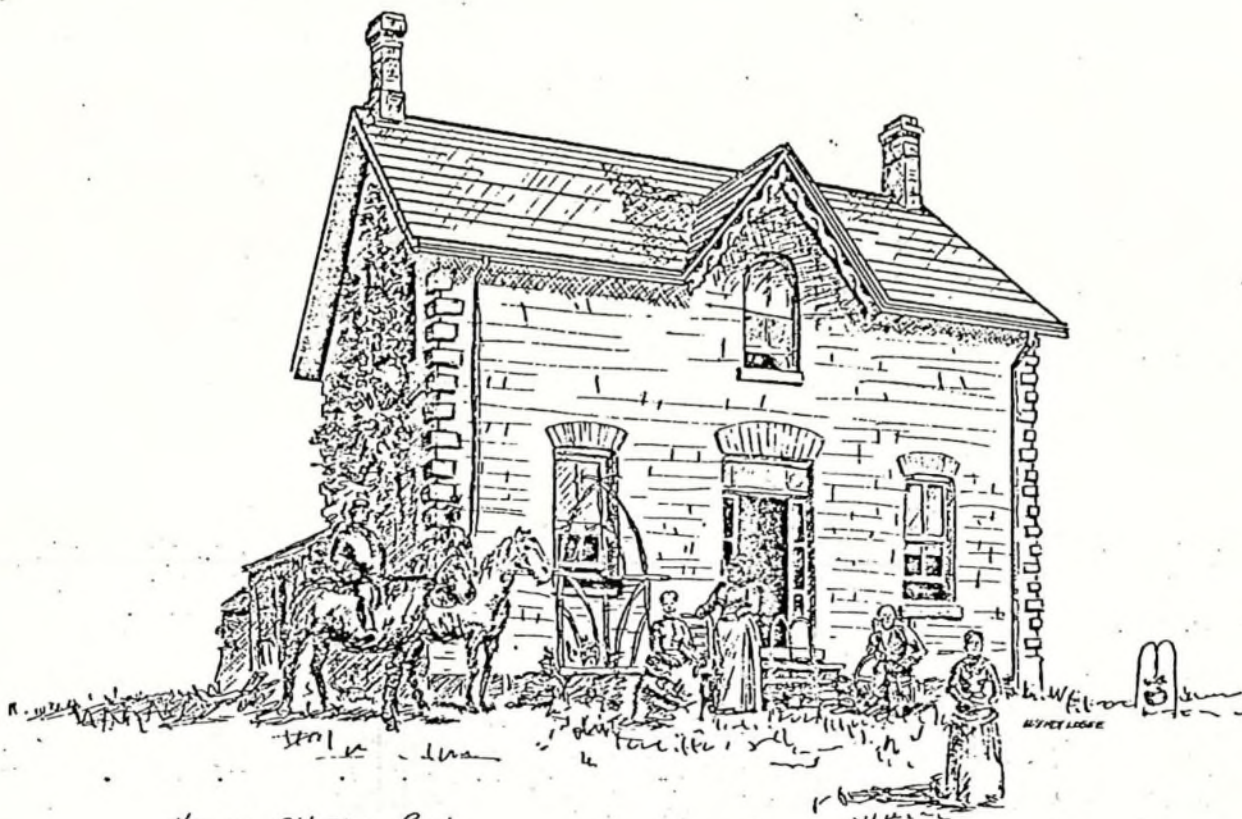
House on Old Stage Road, Lot 10, Concession 4 Built in, 1851
