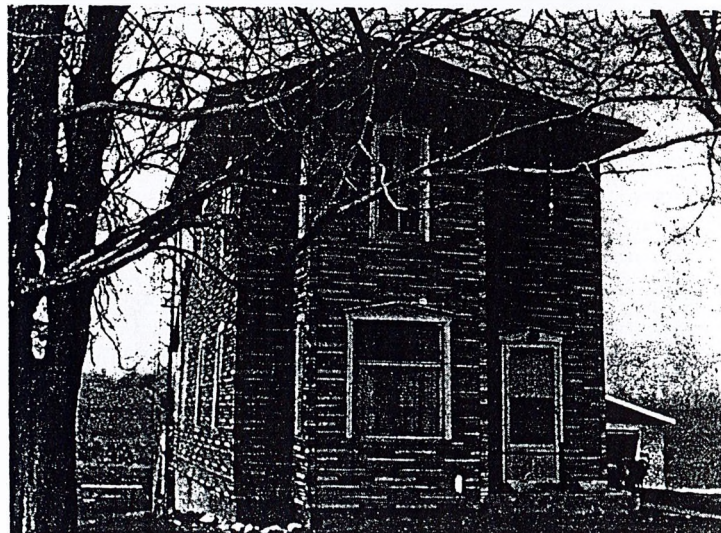
Kosy Kot, the house Aimee's father built after fire had destroyed the first. It originally had a wooden fascia. It is situated one and a half miles west of Salford.
