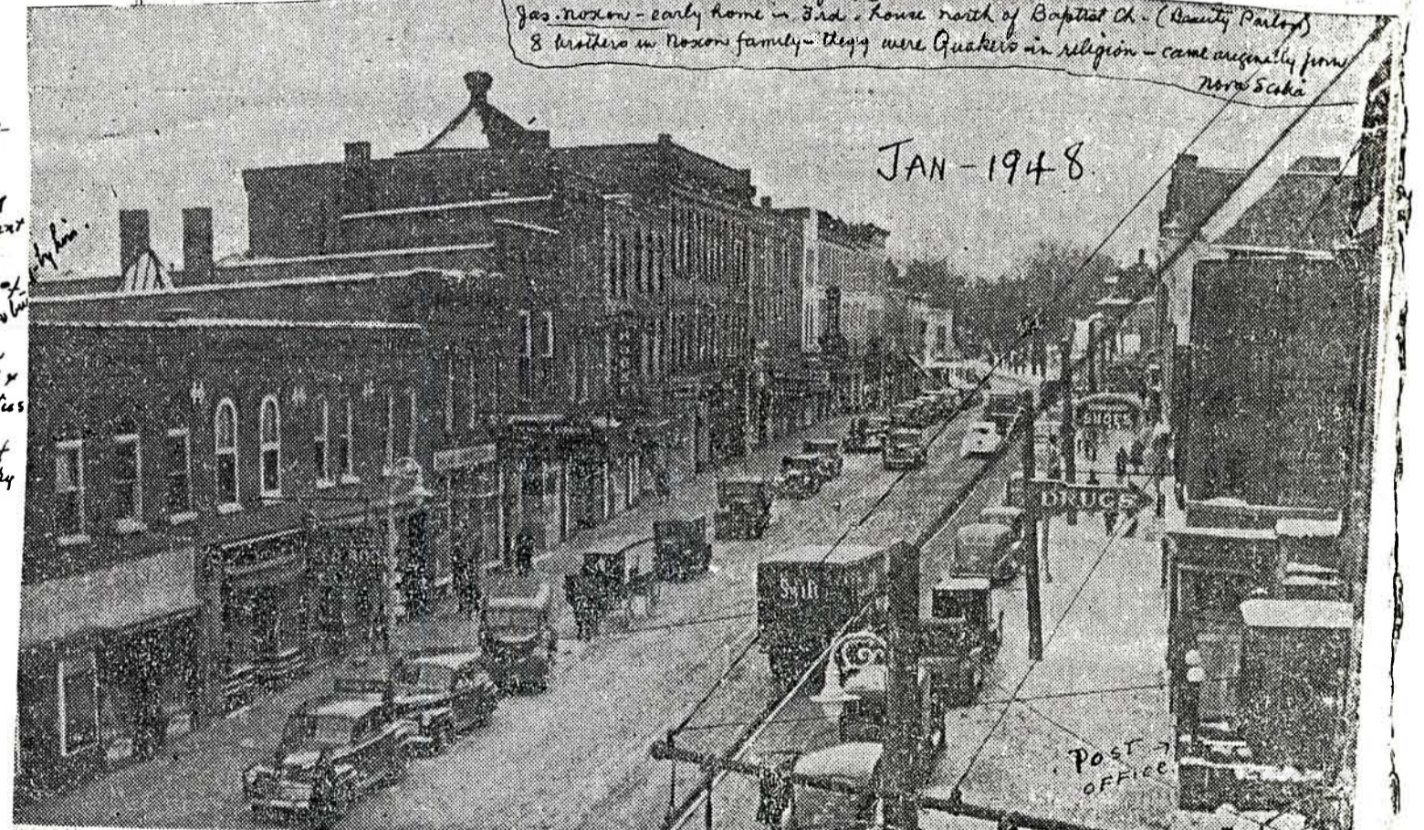
One of the current projects in the Town of Ingersoll is the widening of Thames street, removal of poles and other apparatus restricting a wide open main street through this progressive Western Ontario point. Long famous as the centre of a rich farming and dairy district. Ingersoll is increasing its population, augmenting industrial business and increasing the number of residences. hospital and new collegiate institute are other projects considered by the community.
