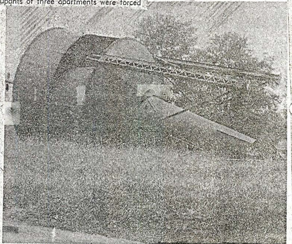
JUNE 1960 END OF THE LINE—A water tower on the CPR line at Ingersoll, near the junction of spur lines leading to Port Burwell and St. Thomas, for years a symbol of the supremacy of the steam engine, toppled in the wake of the CPR's change-over to diesel engines. The tower toppled over after cutting torches sliced through its supports. It will be dismantled and removed. (Photo by Longfield).
