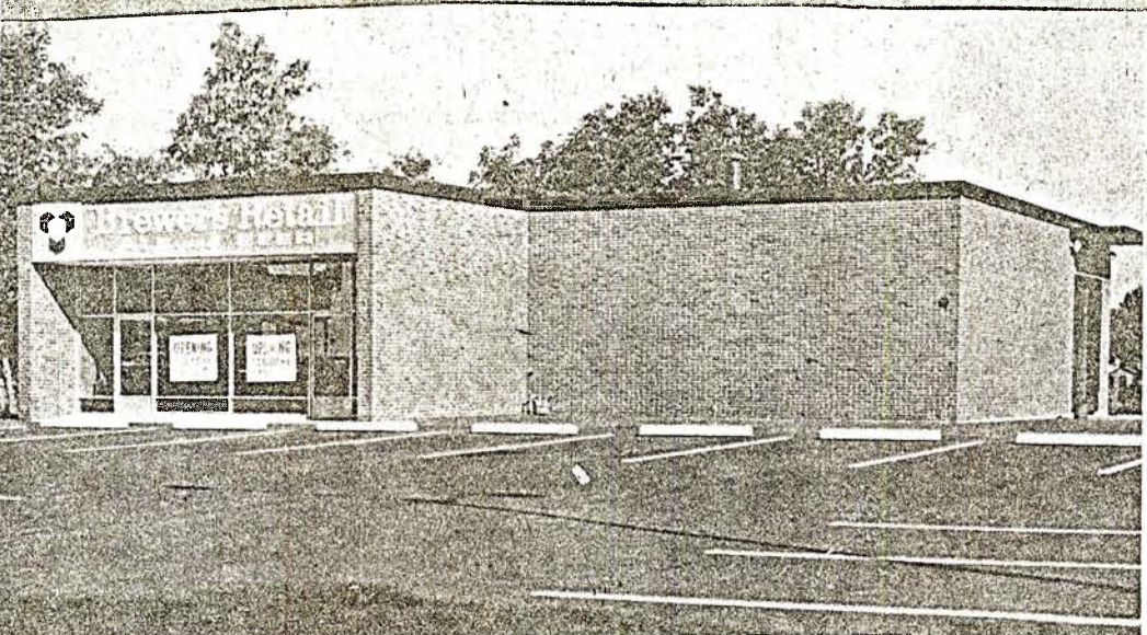
located on Charles Street West the new $65,000 Brewers' Retail outlet is now completed and open for business this week. Aug 8-13-1966
