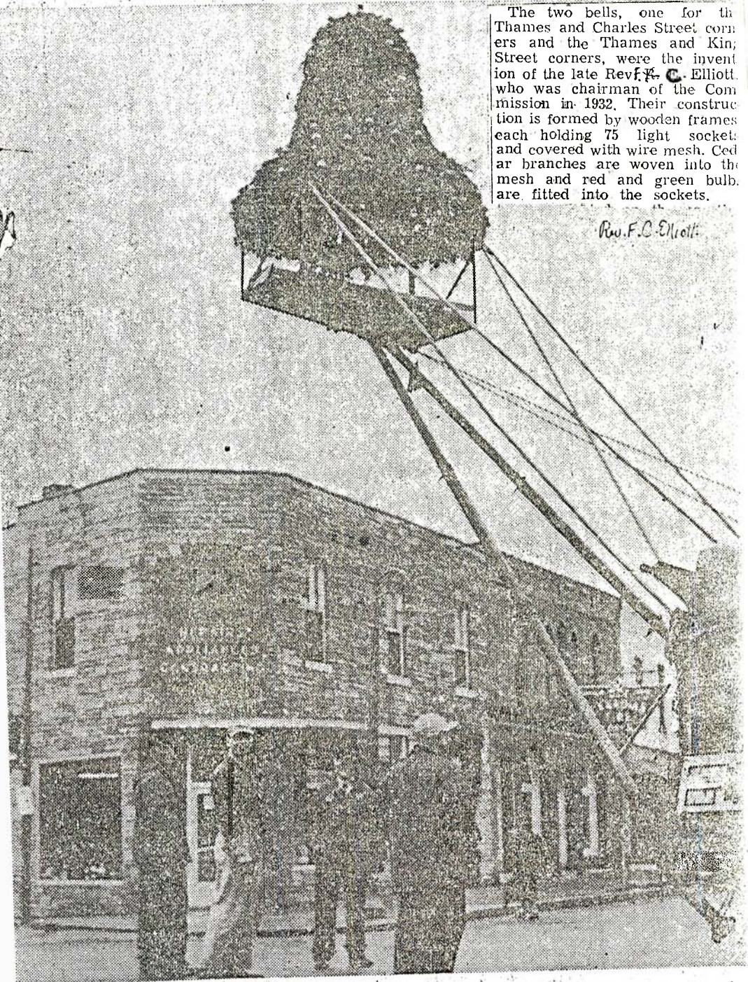
A reminder to Ingersoll residents that Christmas isn't far away is this jumbo-sized bell being hoisted into position over a main intersection in the town. It represents part of the community's "decorate for Christmas" scheme. 1953.
