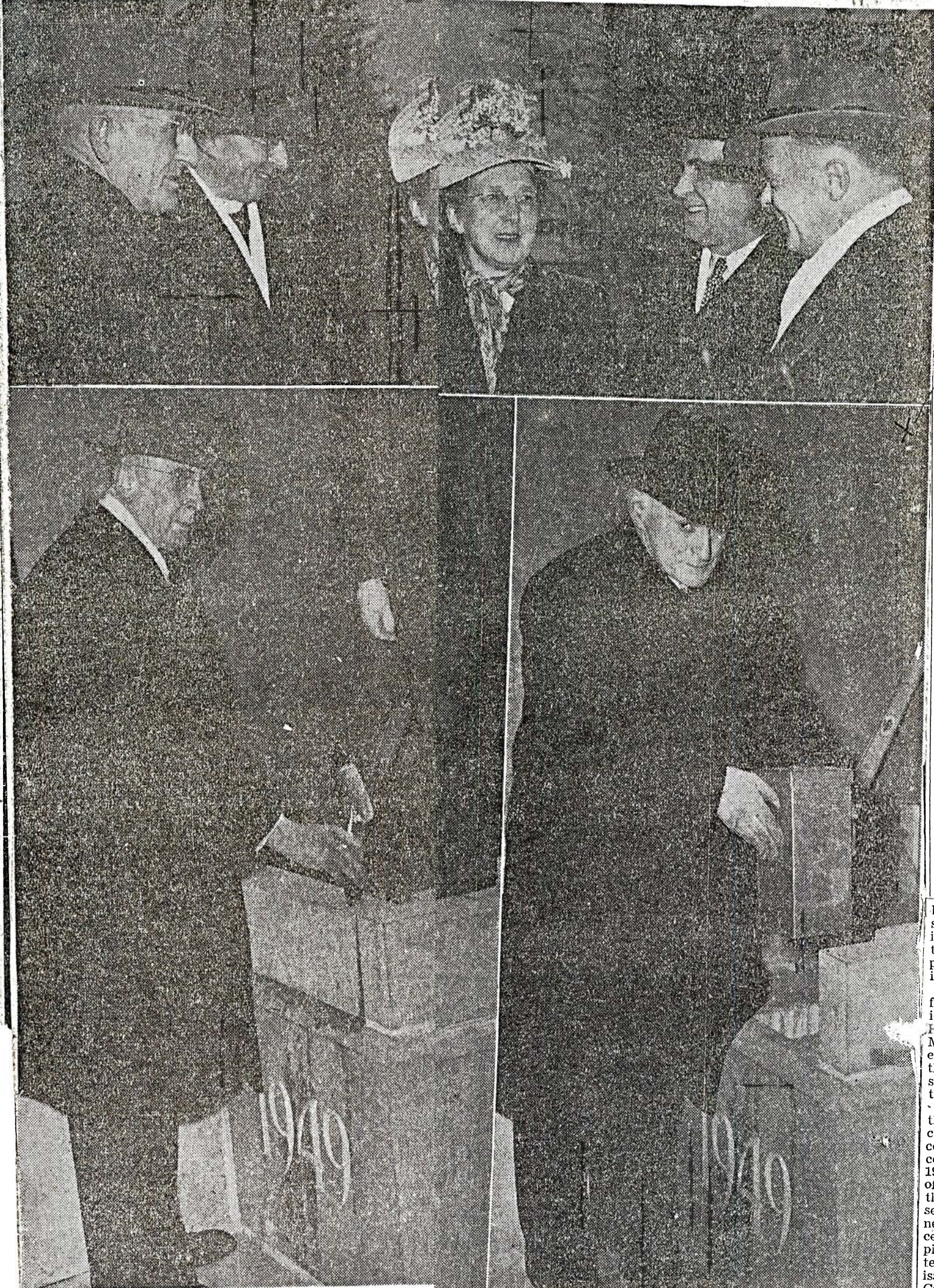
Braving a snowstorm, more than 50 people gathered at the site of the new Alexandra Hospital in Ingersoll yesterday afternoon to watch the laying of the cornerstone. Some of those who took part in the ceremony are seen in the upper photo. From left to right they are: Mayor J. G. Murray, Rev. G. W. Murdoch, Mrs. P. M. Dewar, president of the Women's Auxiliary of the hospital;
