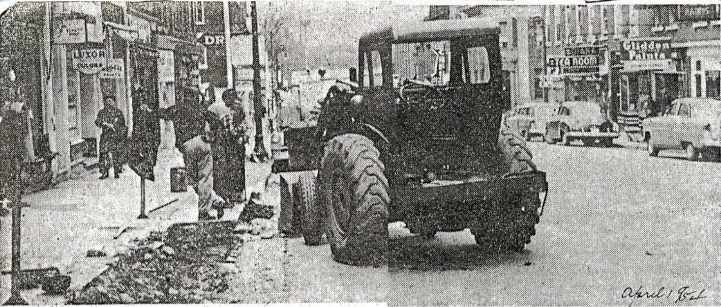
Spring weather has brought a start to another construction boom in Western Ontario. In Ingersoll, workmen are busy tearing up the side of Thames street to make it six feet wider between the Post Office and the Royal Bank. Cost of the job will be $4,500. (Photo by Watmough).
