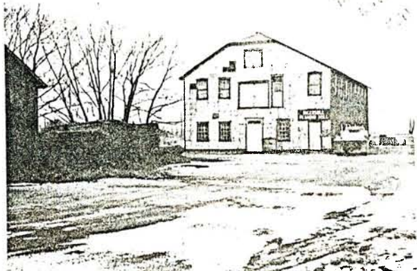
Ingersoll Planning Mill. Nov. 1952 Purchased Feb. 1953 by Smyth & McLeod.
