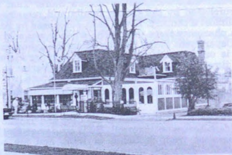
Although the original design of the house is somewhat hidden by more recent porch and patio additions, one can still observe the Mansard style roof on the second storey addition.
