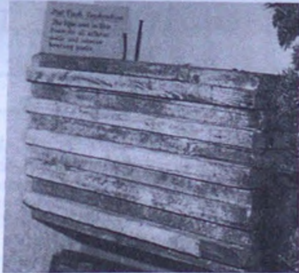
An example of Flat Plank construction original to the Smith House
