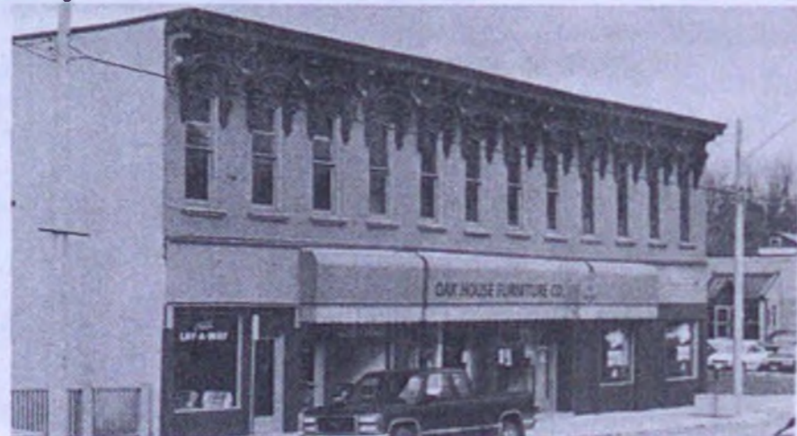
The James McIntyre Building has recently been redecorated to accentuate the Italianate design.
