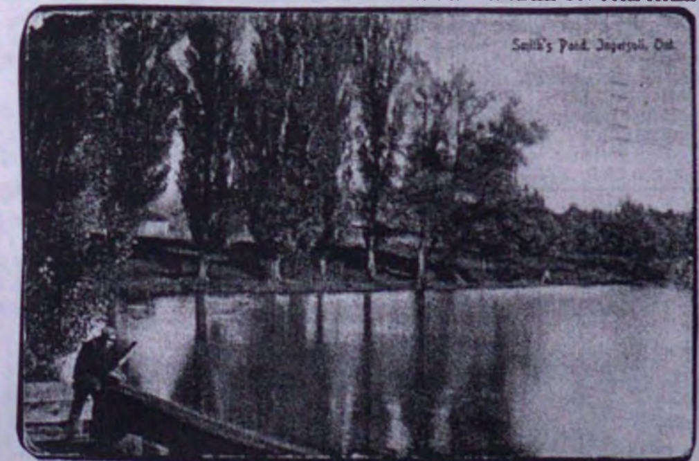
STANDING AT THE DAM LOOKING EAST
