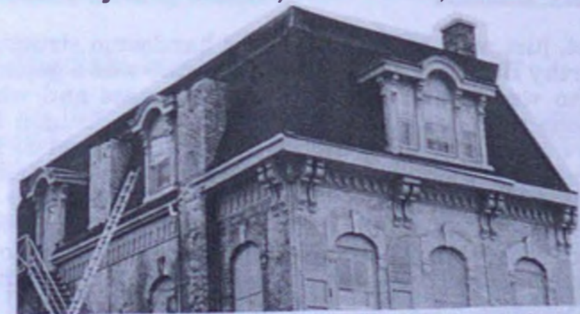
Note the beautiful Italianate features including the Palladian window, wide cornice, detailed brackets and dentils. Also Italianate in design are the toppers on the windows, with keystone accents.
