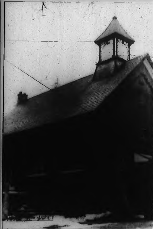
THE OLE' SCHOOL -- This old "one room" school house located, appropriately enough, on Old School Road, is just north of Holbrook and is currently used as a private residence. (Cheryl Clark-Cowan/PHOTO)
